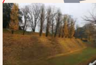
The dry moat and earth work
