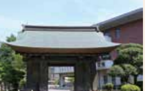
Yakui-mon Gate (Original building)
